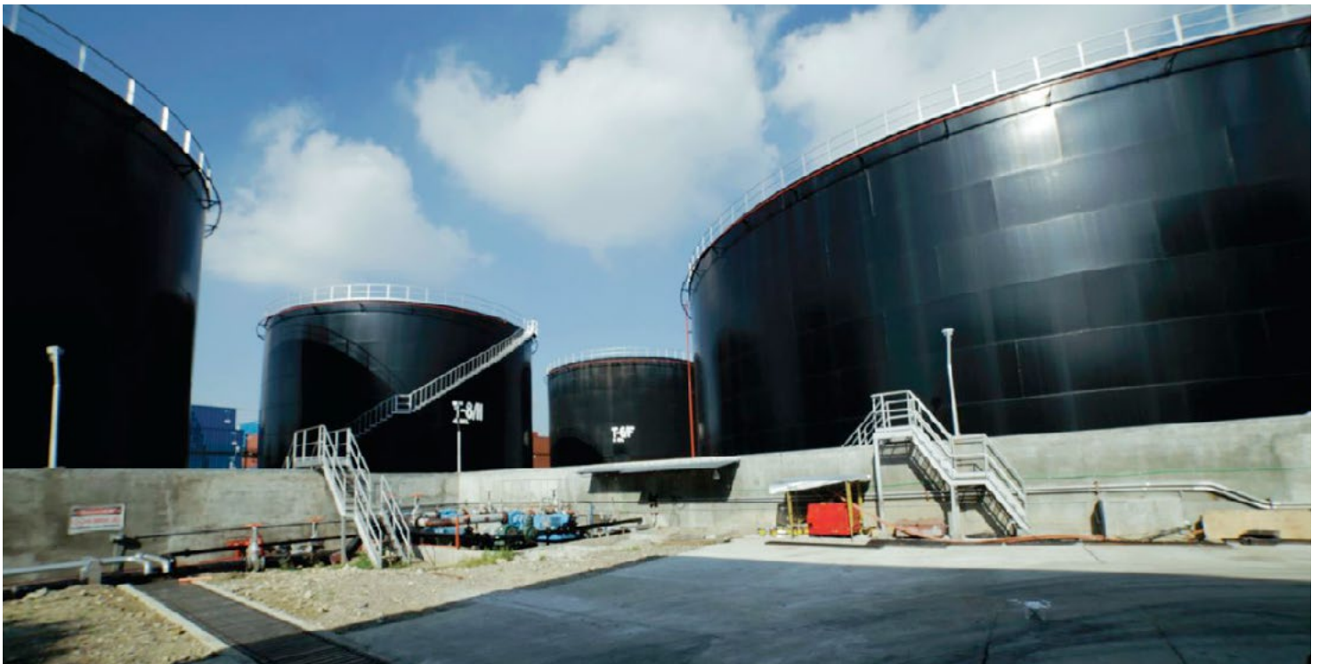
IOC's product storage tanks.
