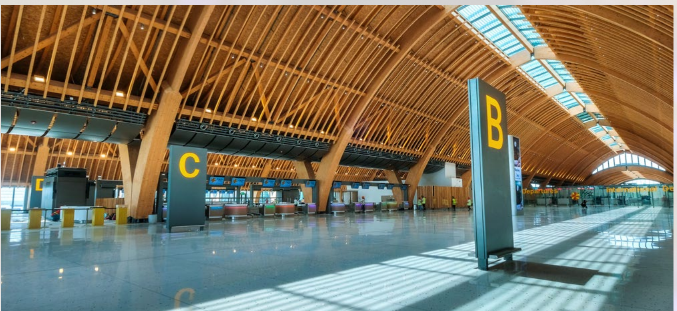
The new Mactan-Cebu International Airport (MCIA) terminal will increase the passenger capacity of MCIA to around 12.5 million. (Photo by Christopher Colinares)
