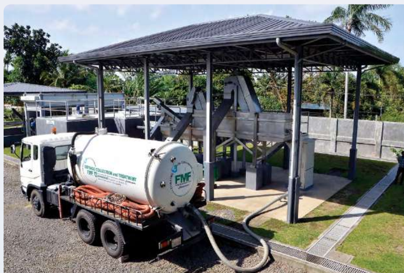
Environkonsult's sludge dewatering facility, sludge holding tank, septage receiving facility, and desludging truck
