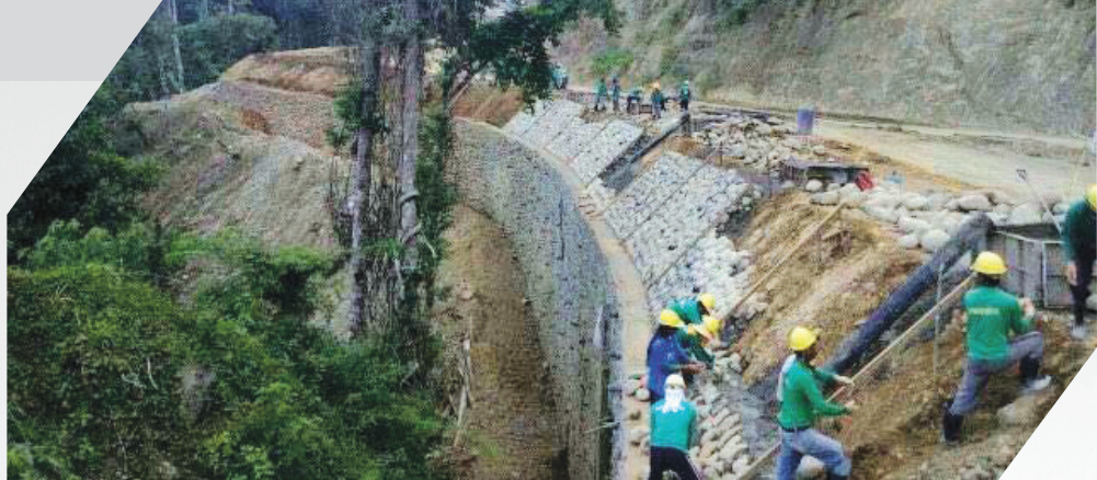
Road works on the Ilagan–Divilacan Road Project
