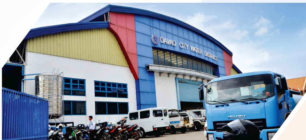
Davao City Water District’s new corporate headquarters
